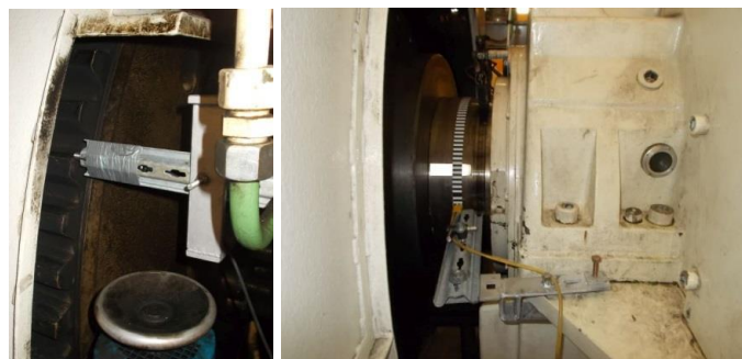
Speed measurements on the engine and on the generator
